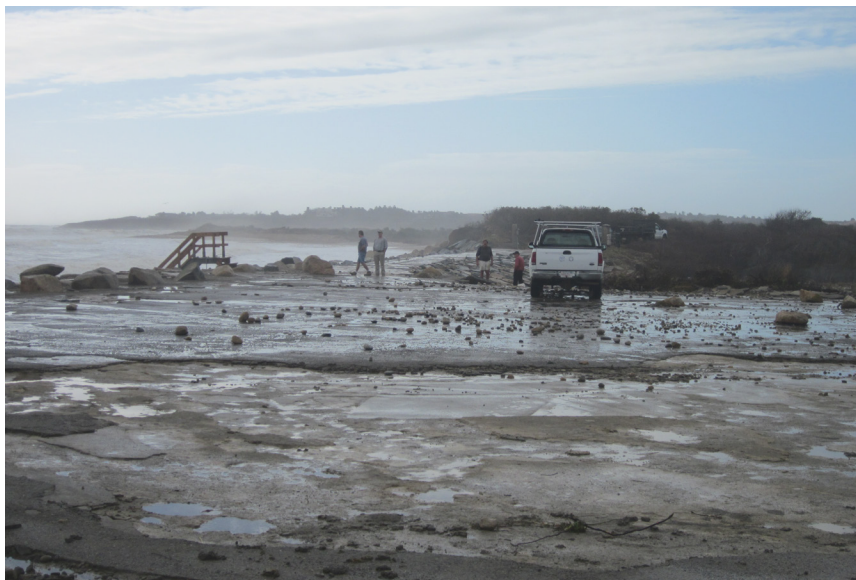
The Squibnocket Beach parking lot following Hurricane Sandy. (Photo by Sara Hoffmann)
